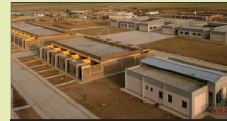
View of houses constructed at Dera Allahyar, Balochistan
