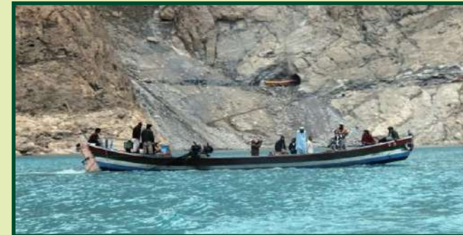
View of ongoing KKH tunnel work site
